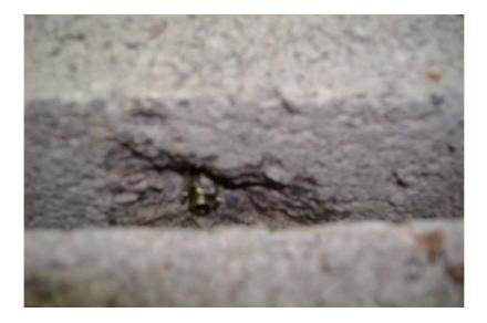
Plate 2 - Showing Rear of Cellular Block with Bottom of Fixing
