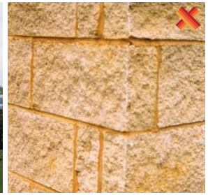
Bad design detail. A cut block slip is used for the corner return. Detail is both untidy, and unsightly.
