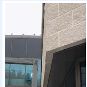
Split faced trough lintel blocks face and soffit (note: cut and bonded joint at 45° trough lintel block)
