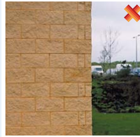
Bad design detail. A cut block slip is used for the corner return. Detail is both untidy, and unsightly.
