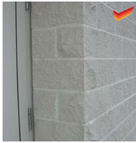
Good design detail. Shows full quoin block return into doorway recess.
