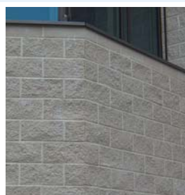
Split faced trough lintel blocks on face (note: cut and bonded joint at 45° trough lintel block)
