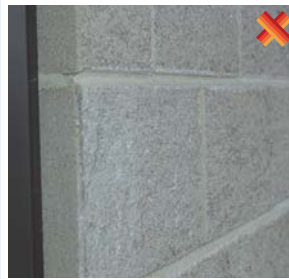
Bad design detail. The ex machine smooth finish of the split faced block has been returned into the recesses. The split faced block could have been ordered with one end shot blasted to add texture to the return face.
