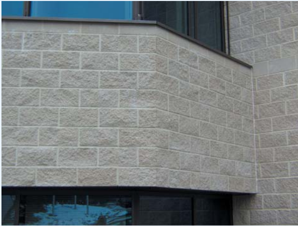
Illustration shows cut and bonded split faced 45° quoin, and quoin trough lintel blocks.
