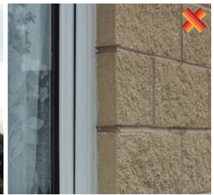
Bad design detail. The ex machine smooth finish of the split faced block has been returned into the recesses. The split faced block could have been ordered with one end shot blasted to add texture to the return face.
